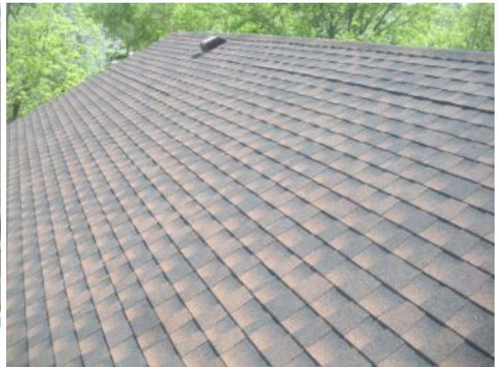
Right side of the house
